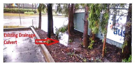
Plate 1: Photograph showing flow moving along an existing drainage swale along the northern boundary of the subject site (image provided by Blueview Pty Ltd, sourced from public submission objection (29/06/2020)
