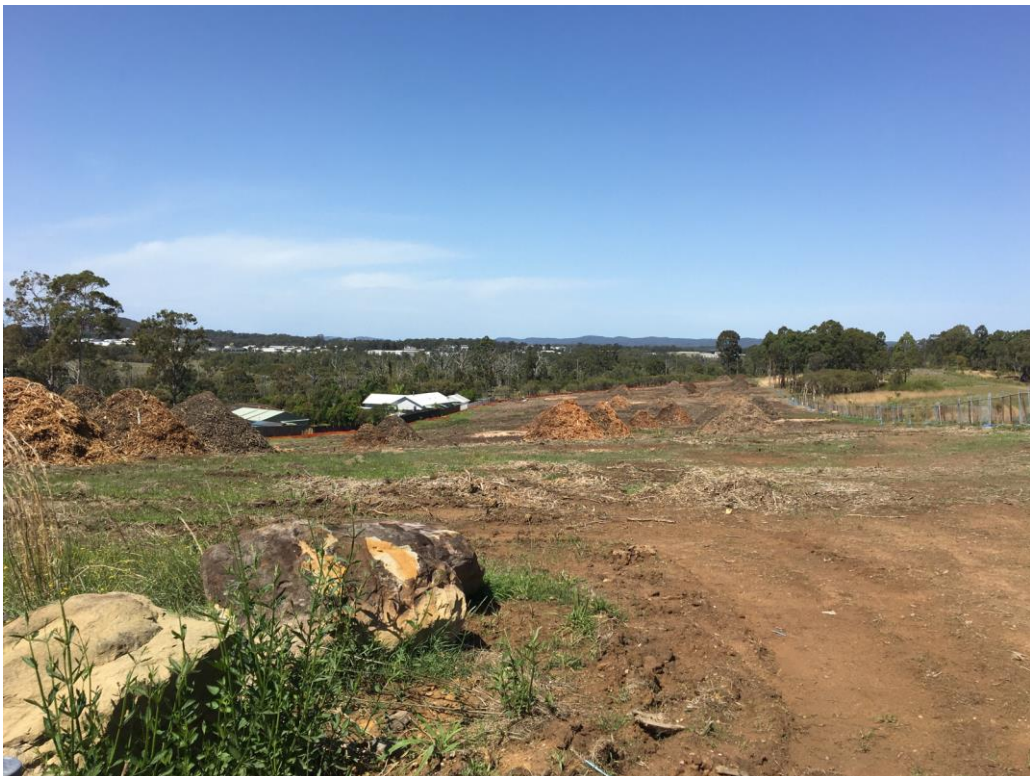
Figure 4: Photograph 15/10/2021 – Viewing Sth from Intersection of Rd 01 & Road 02
