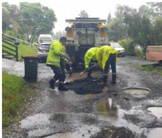
Image: Pothole repair using cold mix which is used to temporarily repair potholes during wet conditions.
