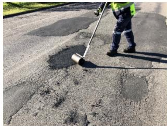
Image: Pothole repair using hot mix, which is used to repair potholes once conditions have dried out and results in a more permanent treatment.
