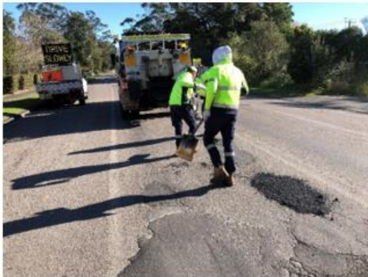
Image: Pothole repair using hot mix, which is used to repair potholes once conditions have dried out and results in a more permanent treatment.
