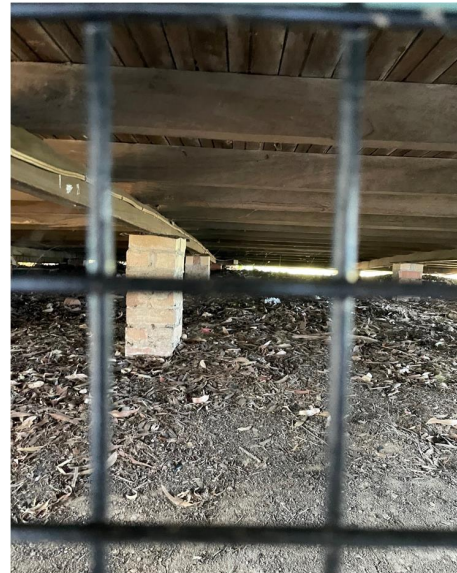
Underside of floor. Bearers and joists unaffected. Floor boards blackened.
