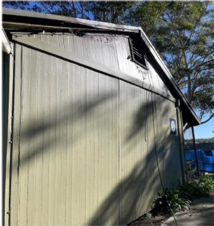
Figure 3: Western elevation of Building Five shown bowing outwards
