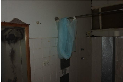
Figure 23 – View within south bathroom, note termite nest.
