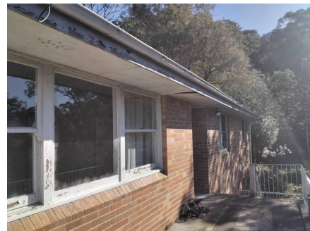
External:Roof - Eaves - Fibro
