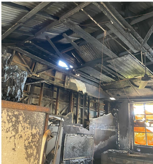
Internal view at east end showing roof and wall framing severely burnt.
