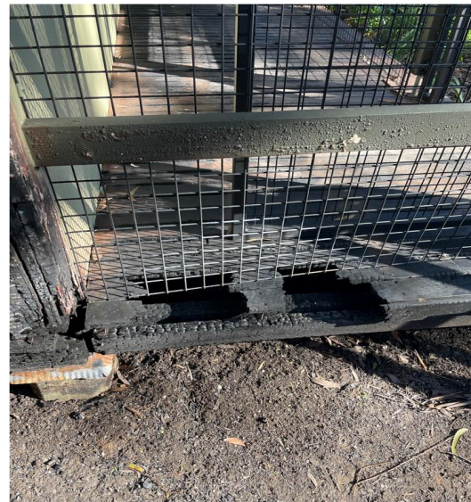
Fire damage to floor at east end.
