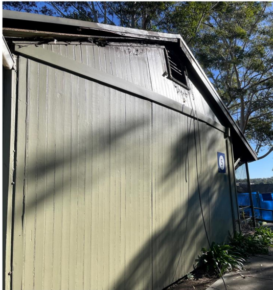
End wall shown bowing outwards.
