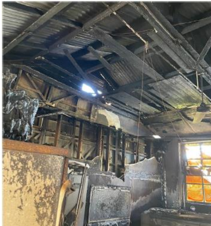
Figure 4: Internal view of east end showing roof and wall framing severely burnt
