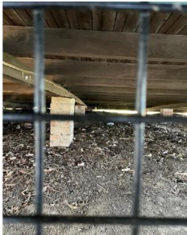
Figure 6: Underside of floor blackened
