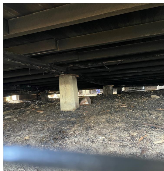
Underside of floor blackened.
