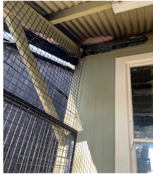
Fire damage to east end wall.
