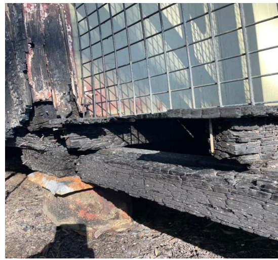
Floor at east end severely damaged.
