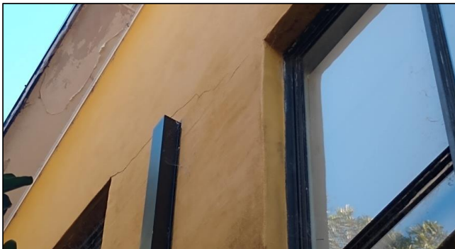
Figure 4: View of the cracked render on the western side of the residence.
