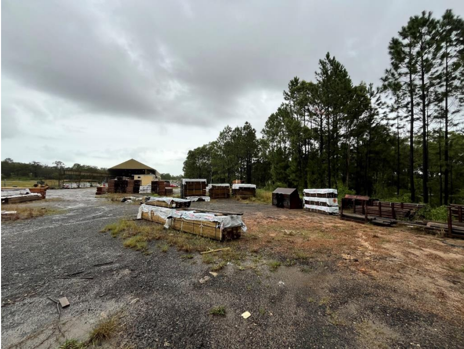
Figure 8: The site looking south west (Source: Site inspection)
