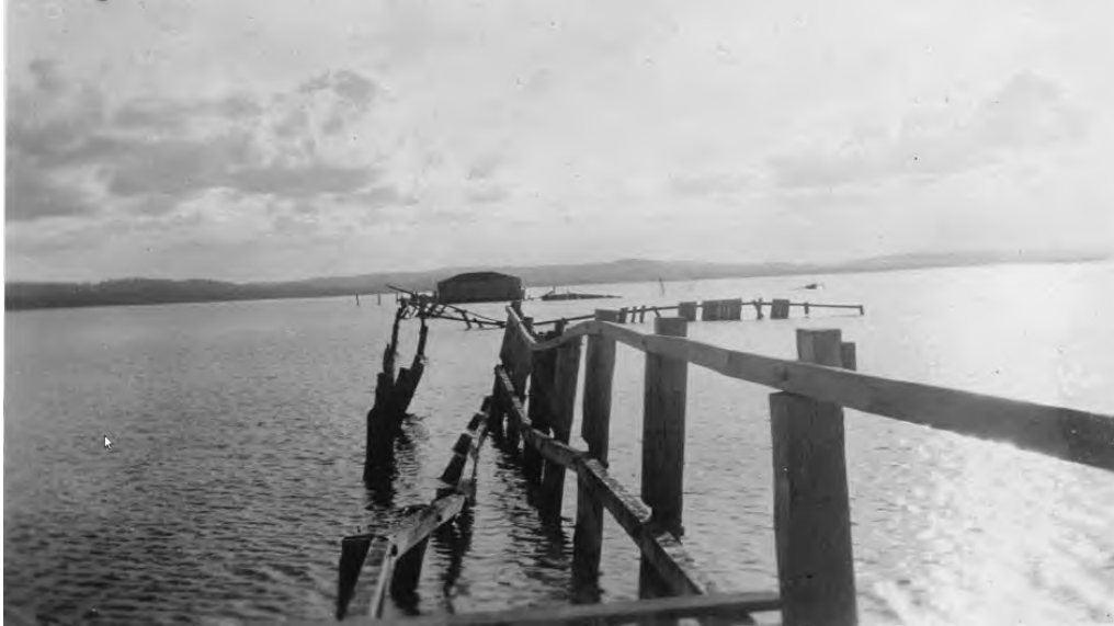
Figure 1.3 Damages to the original Long Jetty (built 1914 by William Henry Price) following flooding in Easter 1927. Courtesy of Central Coast Council
