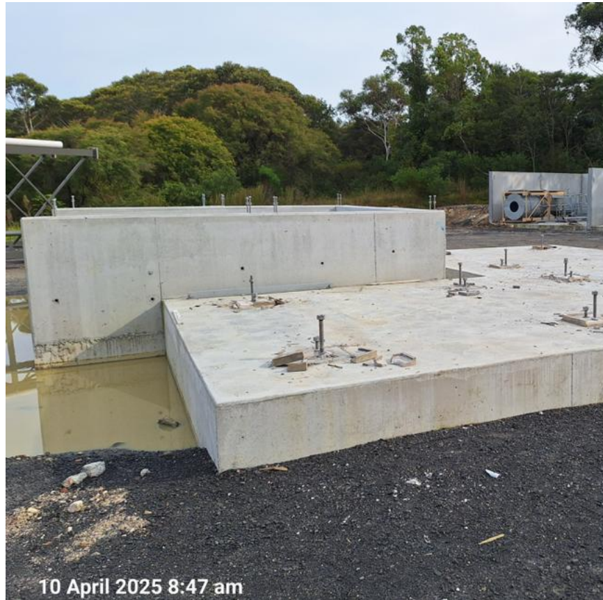
Figure 2-15: View of the concrete slab with silos removed (Source: ATB Morton)
